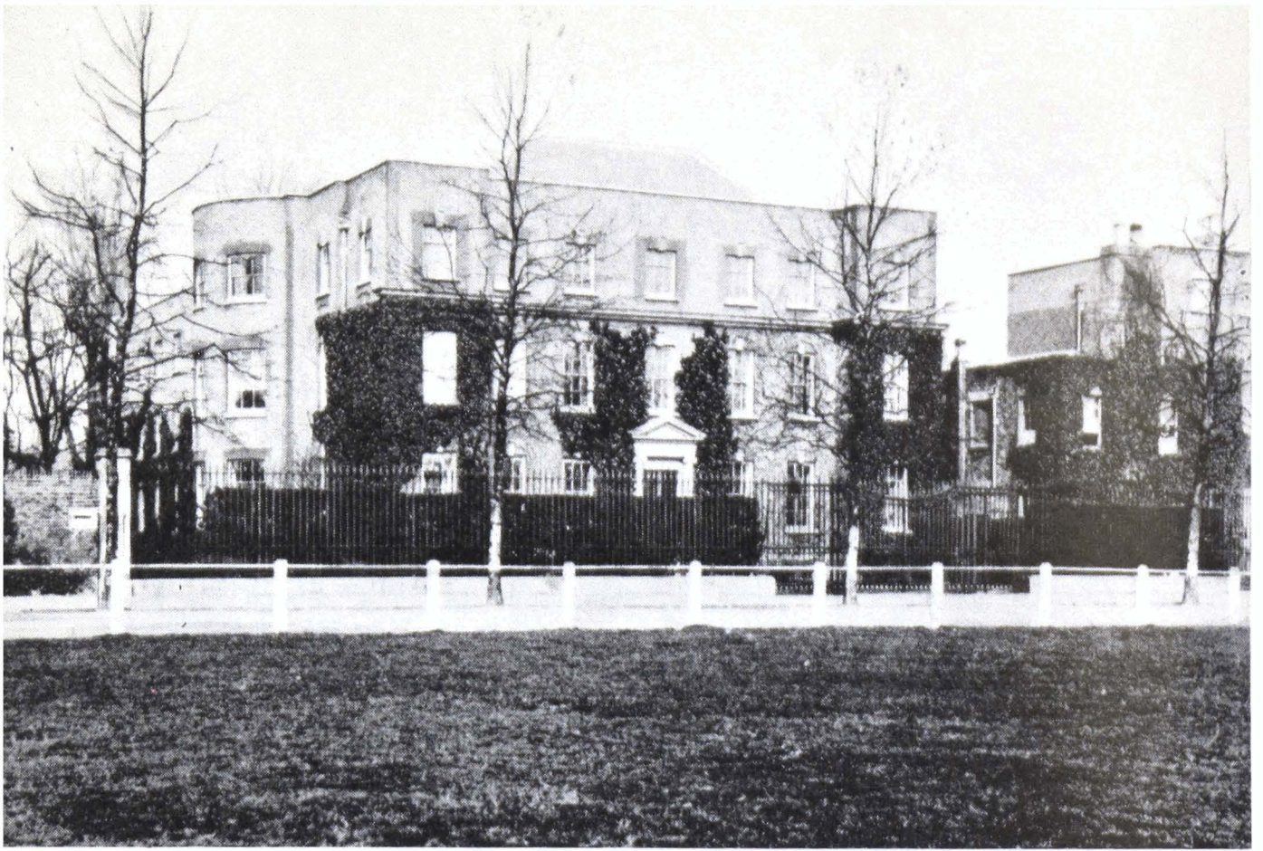
Plate 21 Exterior view of the Herbarium, Kew ( c. 1890), the part that was built during J. D. Hooker's directorship.
